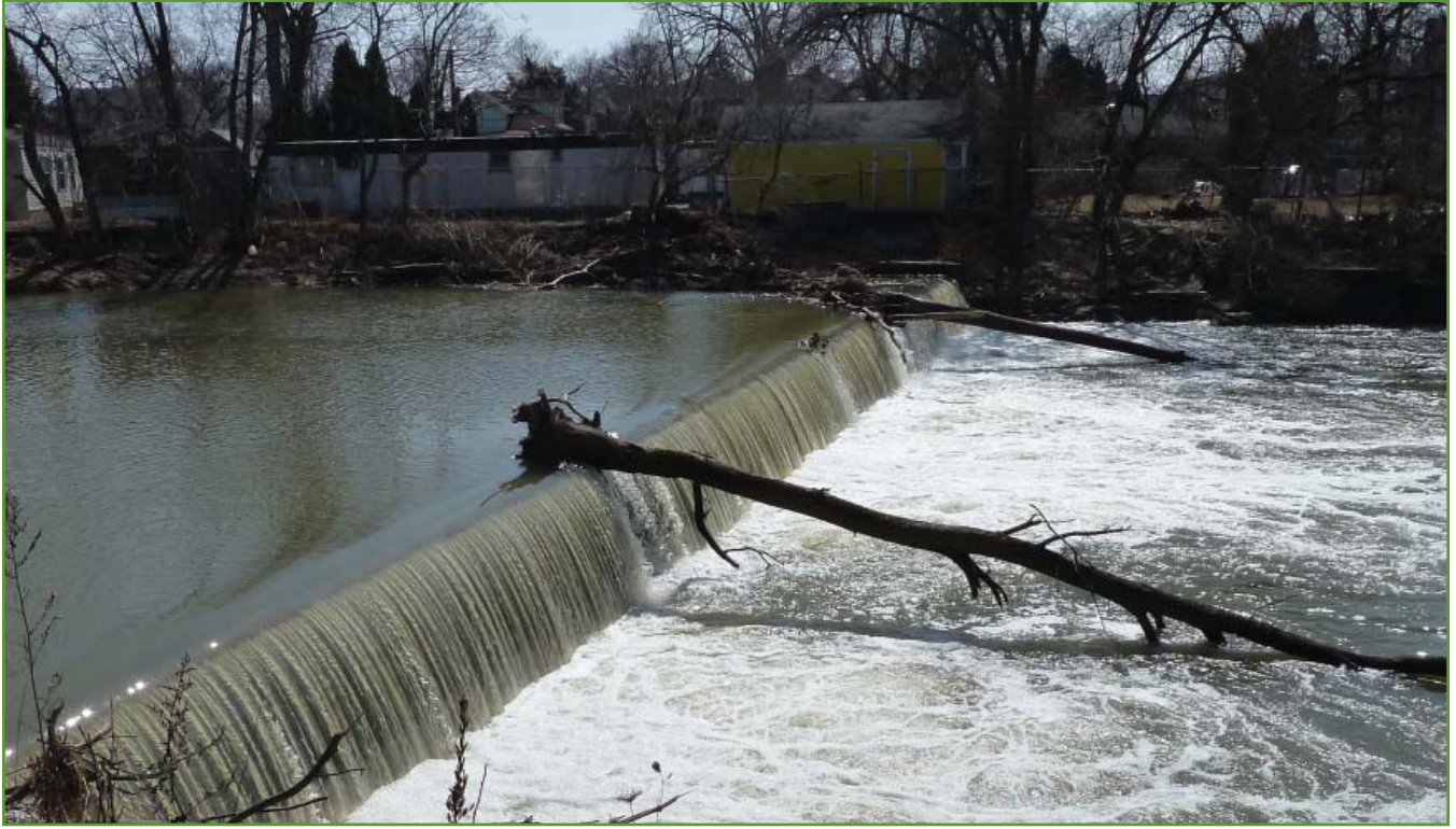
Figure 25. Low head dam, Little River in Huntington, Indiana during normal flow. Photo by USACE taken April 16, 2011.
