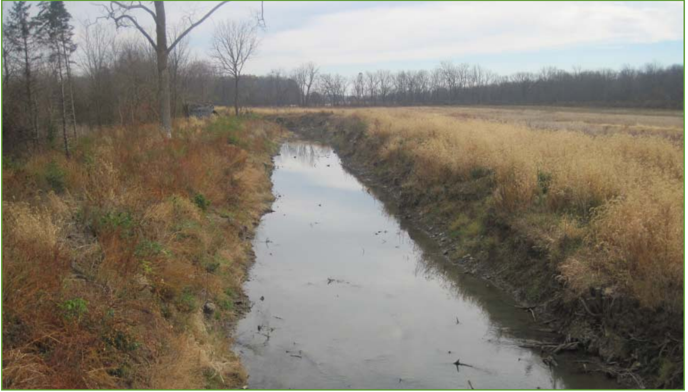
Figure 11. Graham-McCulloch Ditch on November 3, 2010. Photo by USACE.
