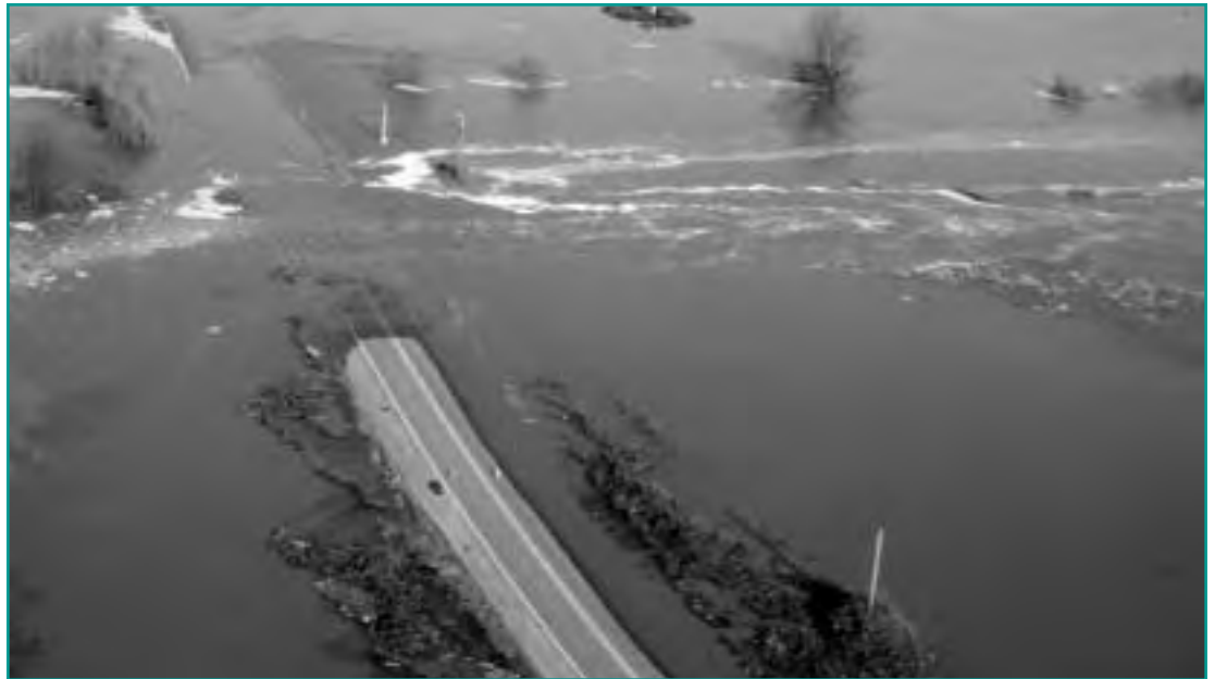
Levee systems provide another method of flood protection. There are over 20 levee systems in the lower Columbia River, and, in high water years, they add another layer of security for residents in flood prone areas.
