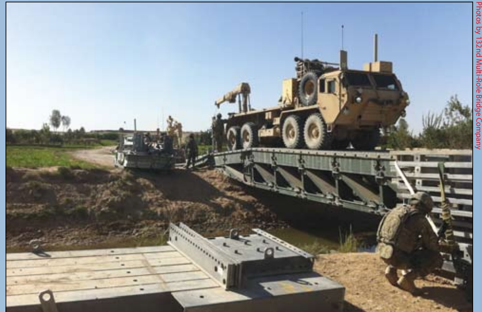
Soldiers from the 132nd Multi-Role Bridge Company (MRBC) work to remove a U.S. Marine Corps Medium Girder Bridge, which was missing parts because of theft, and replace it with a Mabey Johnson Bridge in Helmand province, Afghanistan, in September. Below: Soldiers from the 132nd work on bridges in Urozgan province (bottom), Zabul province (inset left), Kandahar province (inset center left and right) and Helmand province during their current tour.
