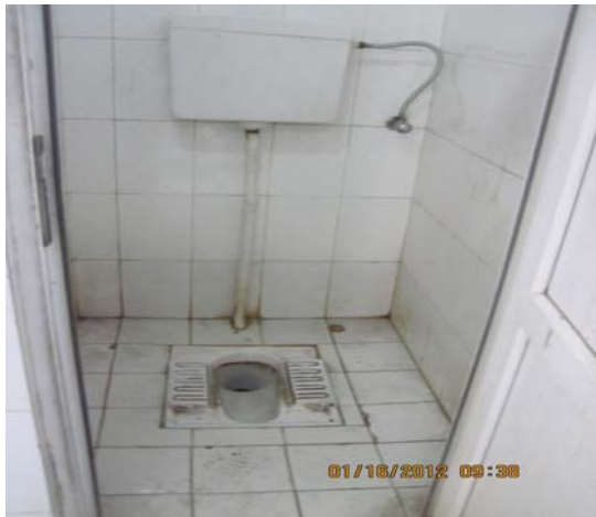
Figure 2 - Eastern Style Toilet in Good Repair in Latrine at Police District 3, Kabul
