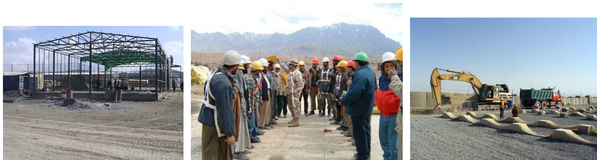
Figure 4. From left: Gym facility being erected at Kabul Military Training Center; Safety training in Pol-e-charki; Digging sewer lines in Kandahar. (Source: USACE – Afghan Engineer District)
