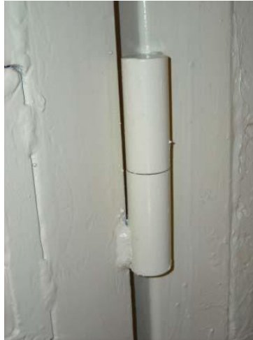
Figure 4. DFIP Hinge
