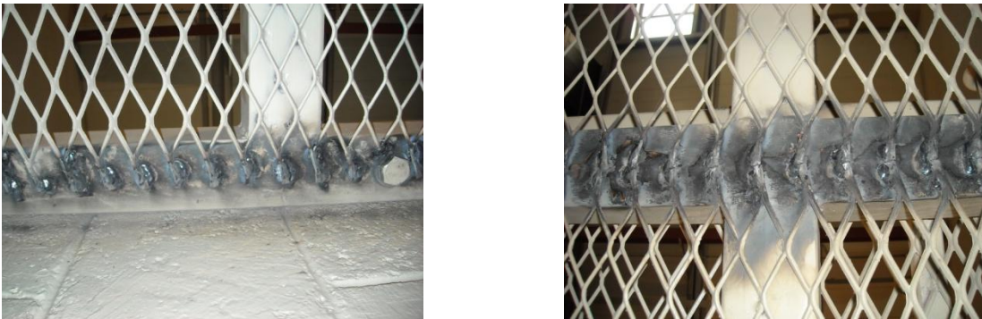
Figure 3. Re-Welded Cell Doors
