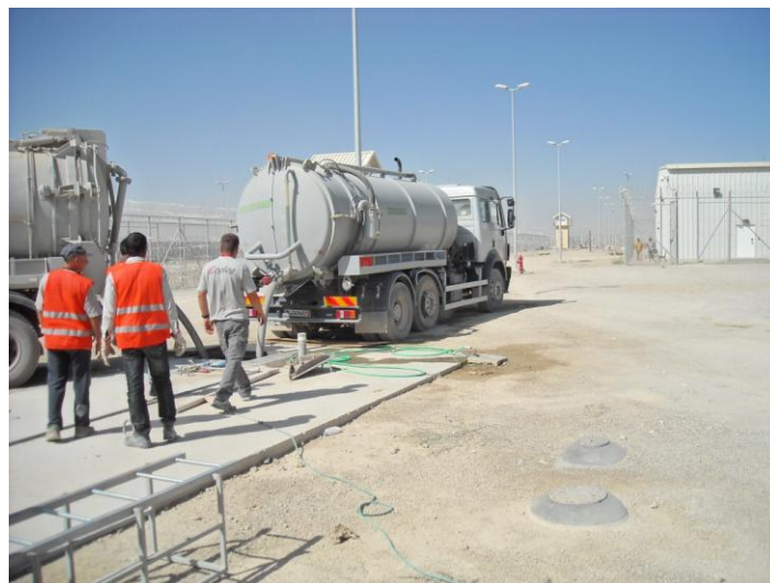
Figure 6. Trucks Collect Sewage
