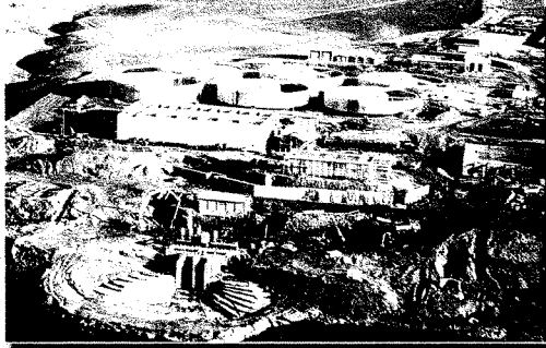
Massive water treatment plant under construction in Erbil, Iraq. The plant was completed in July 2006 and has begun limited operations.
