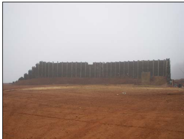
Figure 3-3. Range 3 Main Containment Wall
