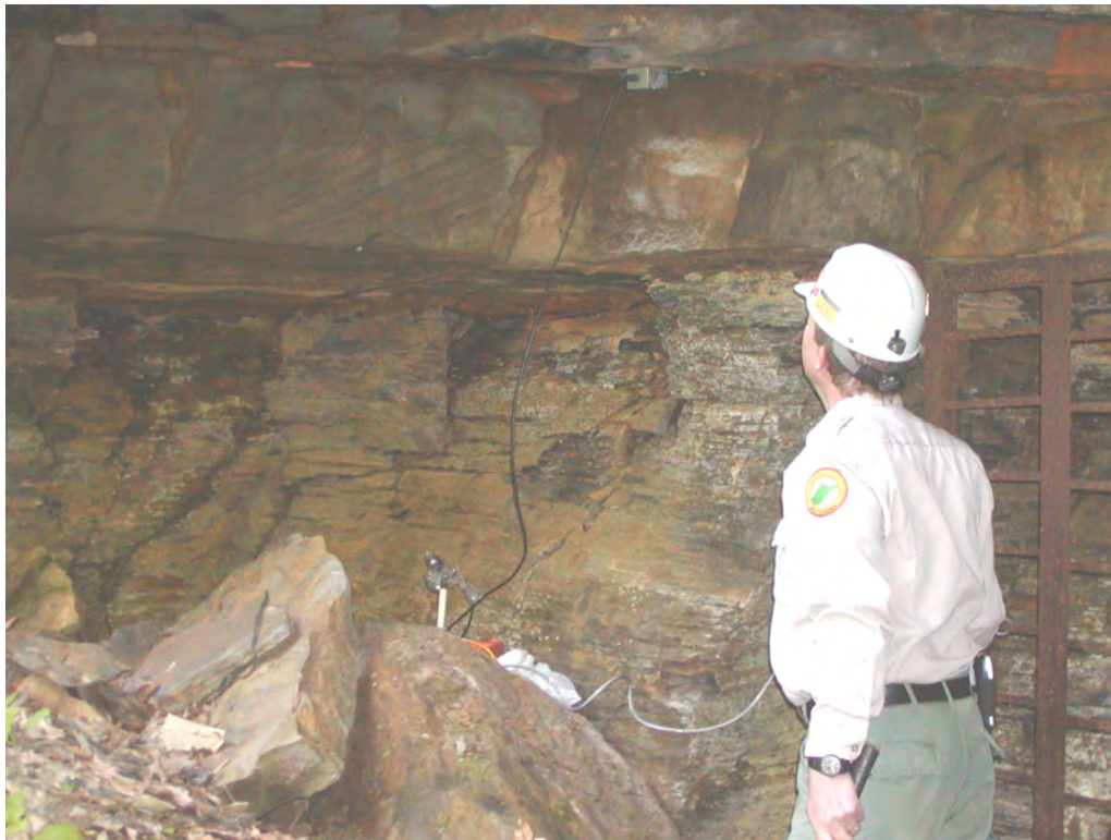
Figure 5. Geophone Bolted to Roof of Portal 2D.
