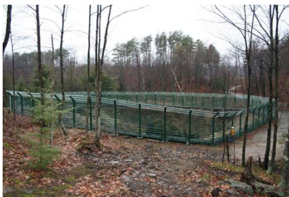
Bat Friendly Closure built by OSM at Glen Lyon Mine Pennsylvania 2007
