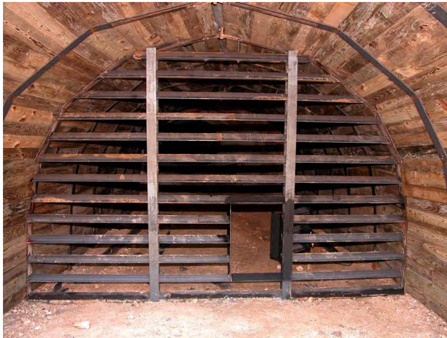
Figure 3. Stabilized mine entrance in Southern Illinois with bat-friendly gate.
