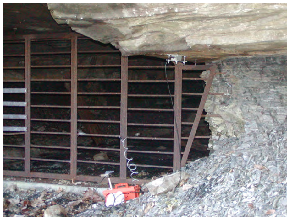
Figure 4. Geophone Bolted to Roof of Portal 2A.
