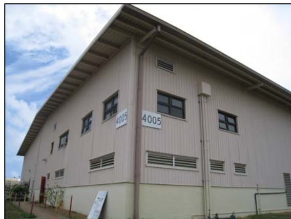
Figure 3-11: Facility 4005 is a storage facility constructed in 1987. Photo taken in July 2009.
