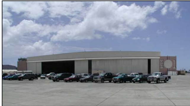
Figure 4-5: Hangar 1. Photo taken May 2004.
