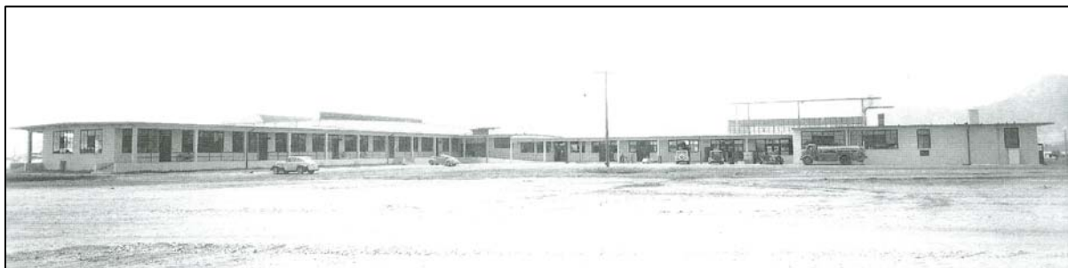
Figure 2-2: Photograph of the Squadron Offices & Storage Building, taken 9 September 1941. Source: National Archives.
