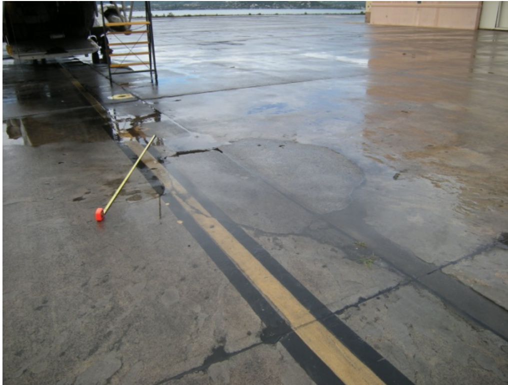
Figure 3-11: Bomb Crater "1" in the center of the photo; radial scars in the lower left corner; the corner of Hangar 1 at the upper right, and the bay in the upper center.
