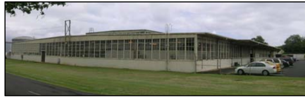
Figure 3-6: Facility 250, note the band of multi-lite, steel frame windows circling the building and the wide overhang of the roof at the loading area on the right. Photo taken in 2003.
