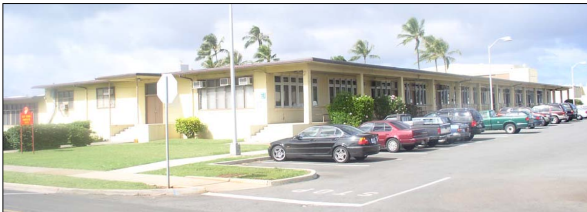
Figure 2-3: Photograph of the Squadron Offices & Storage Building. Photo taken in May 2004.
