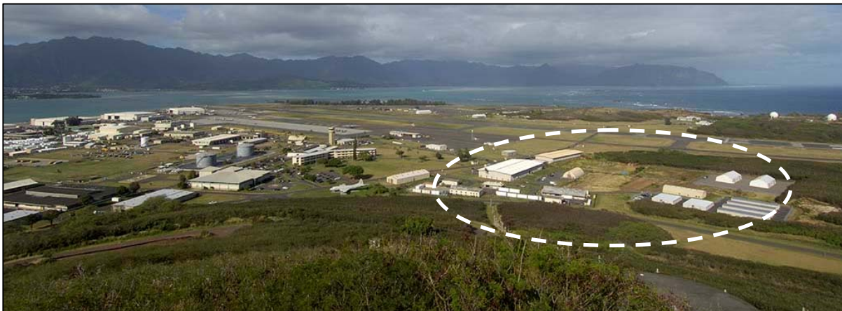
Figure 3-9: Photograph taken from Kansas Tower looking toward the runway. The cluster of storage facilities is visible at the far right. Facility 250 is visible at the far left. Photo taken in 2006 by Franzen Photography.
