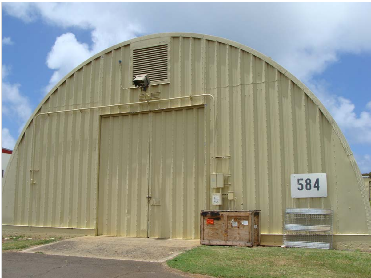
Figure 3-8: Photograph of the facility 584.
