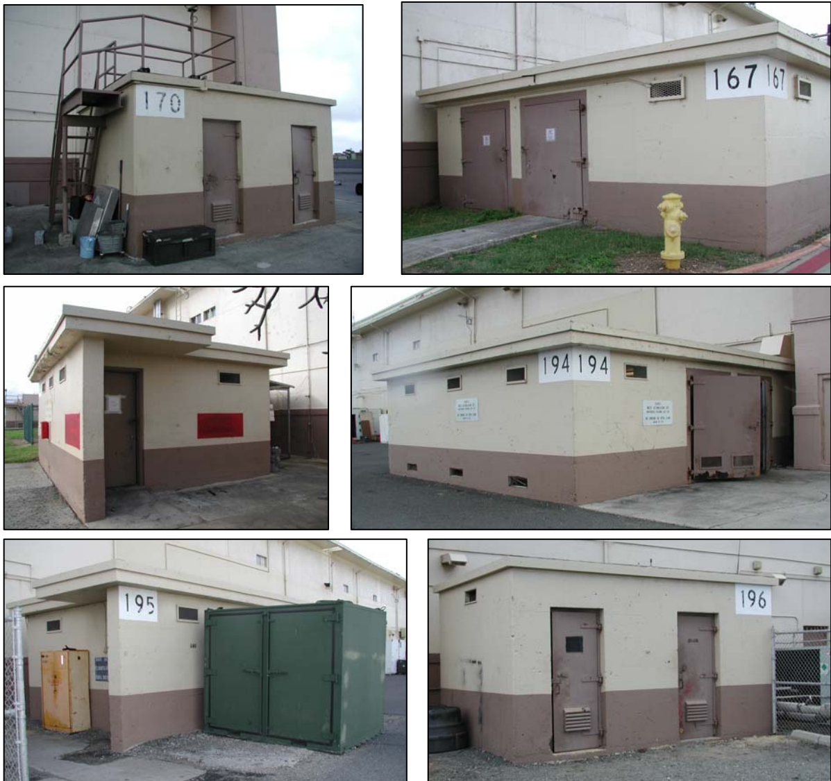
Figure 4-7: Photos above all showing the adjacency to Hangar 1. Top left: Facility 170. Top right: Facility 167. Middle left: Facility 168. Middle right: Facility 194. Lower left: Facility 195. Lower right: 196. Photos taken in 2004.
