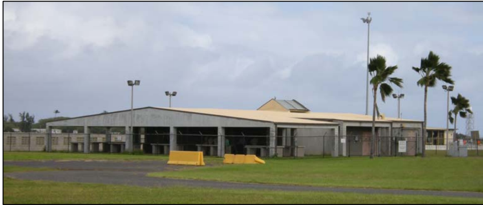
Figure 4-8: Facility 4054. Photo taken in January 2009.
