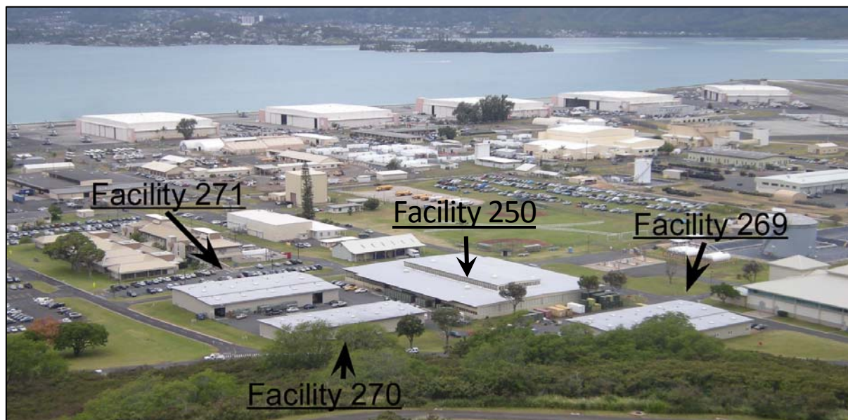
Figure 3-5: Facilities 250, 269, 270, & 271. Photo taken in 1999.
