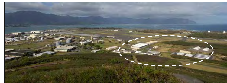
Figure 3-9: Photograph taken from Kansas Tower looking toward the runway. The cluster of storage facilities is visible at the far right. Facility 250 is visible at the far left. Photo taken in 2006 by Franzen Photography.
