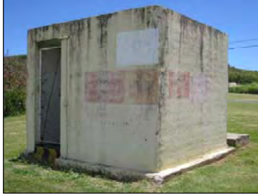
Figure 8-6: Facility 995. Photo taken in 2009.
