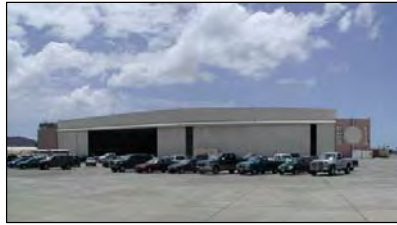
Figure 4-4: Hangar 1. Photo taken May 2004.
