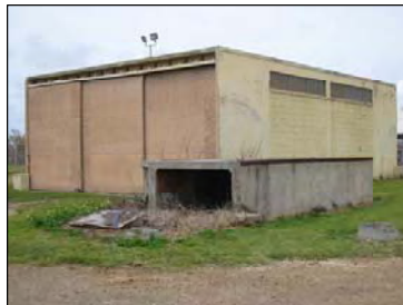
Figure 8-3: Facility 602. Photo taken in 2009.
