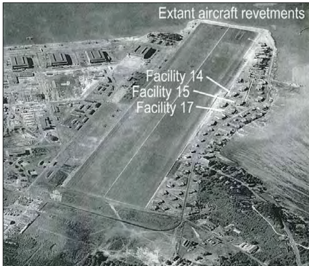
Figure 8-2: Photograph dated November 16, 1943 showing the revetments alongside the landing mat. South at top. Source: National Archives.
