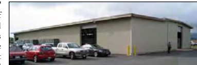
Figure 3-7: Facility 271. Photo taken in April 2009.
