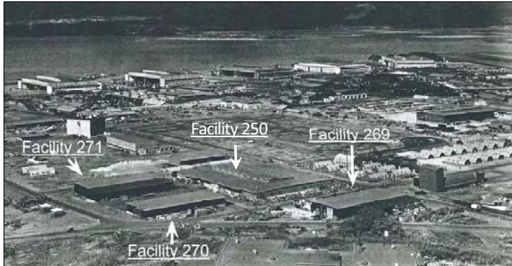
Figure 3-4: Photo dated August 26, 1945 showing Facilities 250, 269, 270 & 271 shortly after they were built. Note the additions along the long sides of Facilities 271 and 269. In the original photo it is not clear if these are already enclosed additions or just roofed over open air areas. Source: - National Archives.
