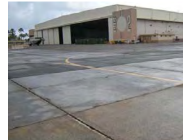
Figure 25: Damaged Area "j," pitted and repaired areas in the center and lower left of the photo. Photo taken looking east, toward Hangar 2.
