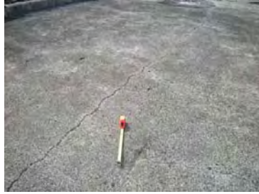
Figure 28: Damaged Area "k," apparent bullet impact mark in Seaplane Ramp 3. Photo taken looking south, toward the bay.
