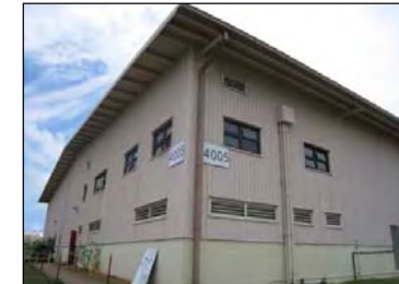
Figure 3-11: Facility 4005 is a storage facility constructed in 1987. Photo taken in July 2009.
