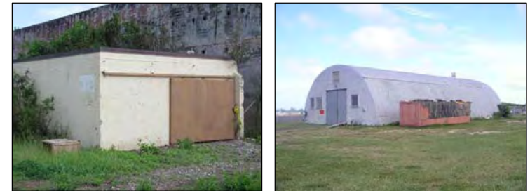
Figure 8-5: Left: Facility 612. Right: Facility 620. Photos taken in 2009.
