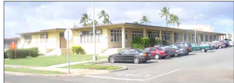
Figure 2-3: Photograph of the Squadron Offices & Storage Building. Photo taken in May 2004.
