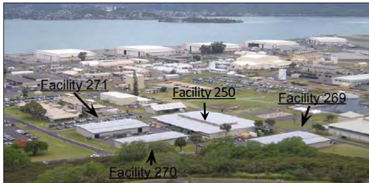
Figure 3-5: Facilities 250, 269, 270, & 271. Photo taken in 1999.
