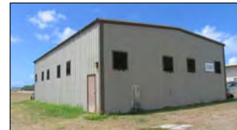
Figure 3-10: Facility 5068 is a balancarbon reclamation facility constructed in 1991. Photo taken in August 2009.
