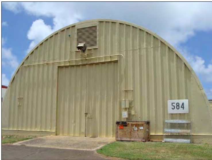
Figure 3-8: Photograph of the facility 584.
