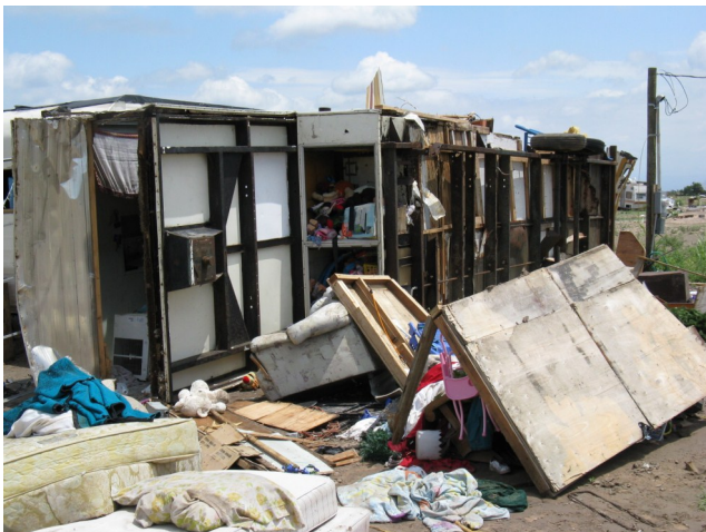
Flipped/Destroyed trailer home, Alton, TX, May 16, 2008
