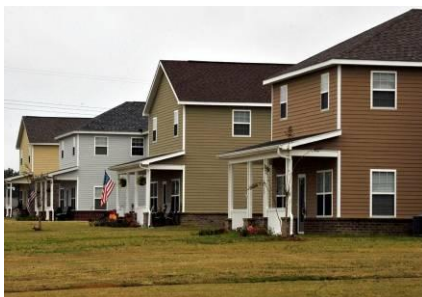
Family Housing at Moody AFB, Georgia
