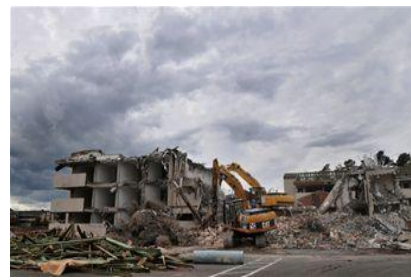
Demolition of old dorms
