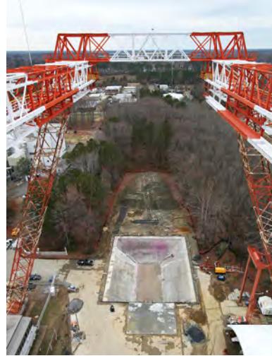
A 2011 aerial view of the Hydro Impact Basin.
