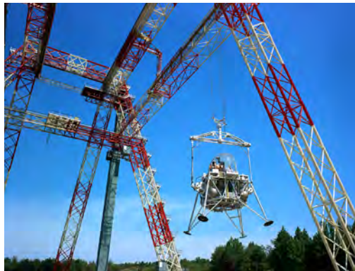
A 1965 LEM suspended from the Gantry.
