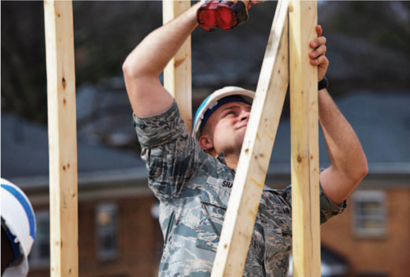
A member of Vet Corps rebuilds a house.
