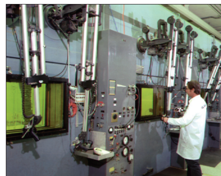
Irradiated targets are transported to TA-48 for chemical processing within a bank of hot cells that are shielded by 20 inches of concrete.
