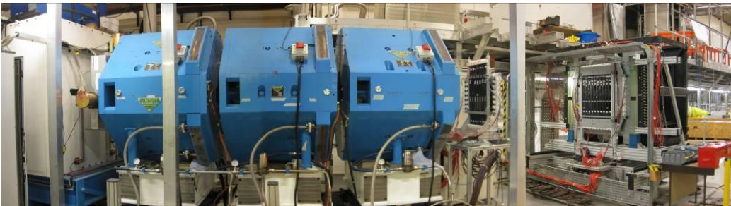
Figure 7: Photo of elements downstream of Decay Solenoid Area: Q7, Q8, Q9, TOF1, TOF2, KL, and part of EMR.
