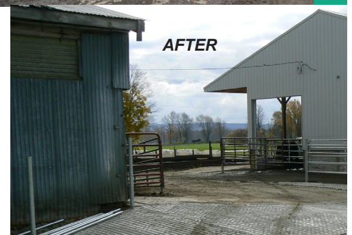
Slated concrete allows for the control of animal waste and sediment runoff. (Different angle)
