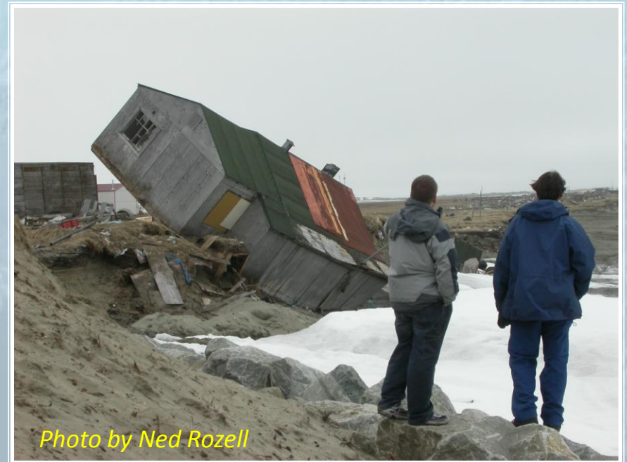
Coastal erosion.... October 2005
