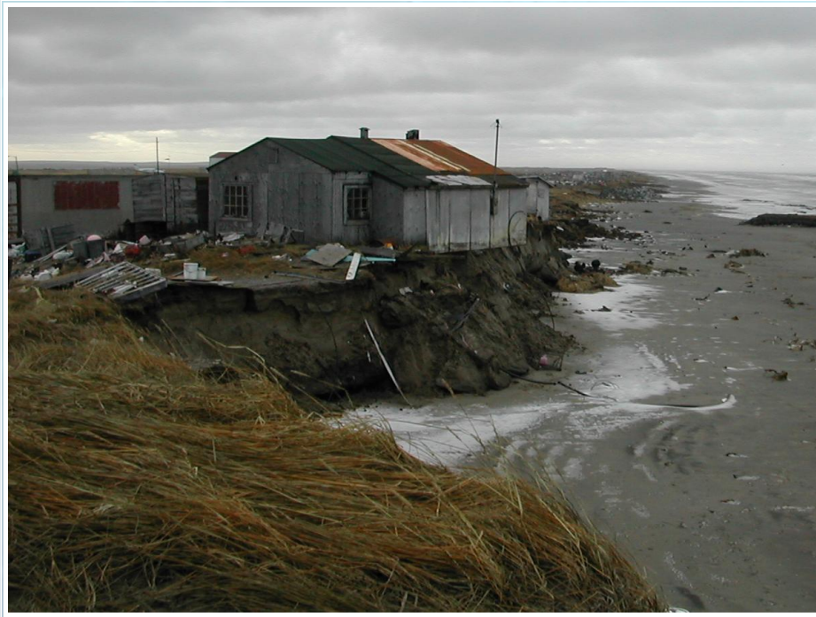
Coastal erosion.... October 2004
