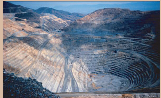
Visible from space, the Bingham Canyon copper mine in Utah has produced more than 12 million tons of porphyry copper. The mine is more than 4 kilometers (2.5 miles) across at the top and 800 meters (0.5 mile) deep and is one of the engineering wonders of the world. Photograph by C.G. Cunningham, USGS.
