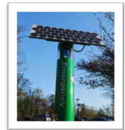
Copper wiring provides a reliable conduit to power emergency lighting systems.
