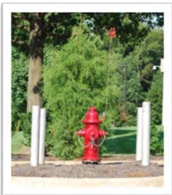
Iron and steel used in guard posts provides a strong barrier.
