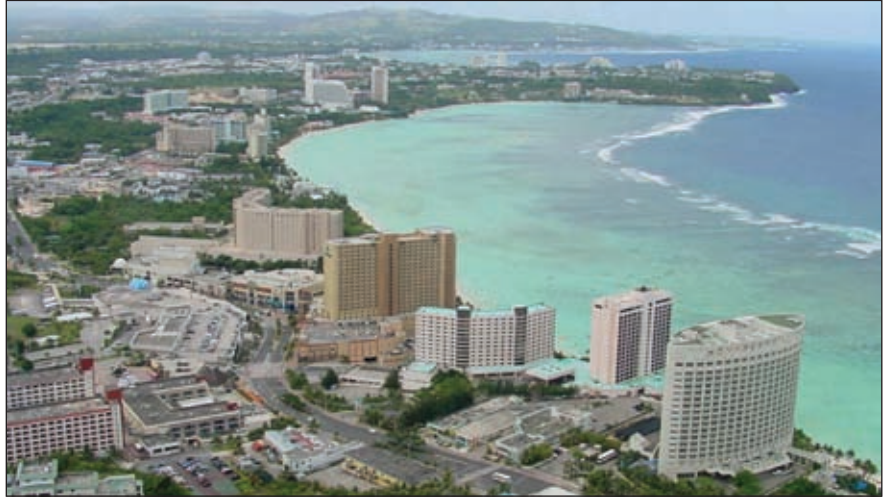
Figure 15.7. High density development along the TBMP. Photo: J. Jocson.
