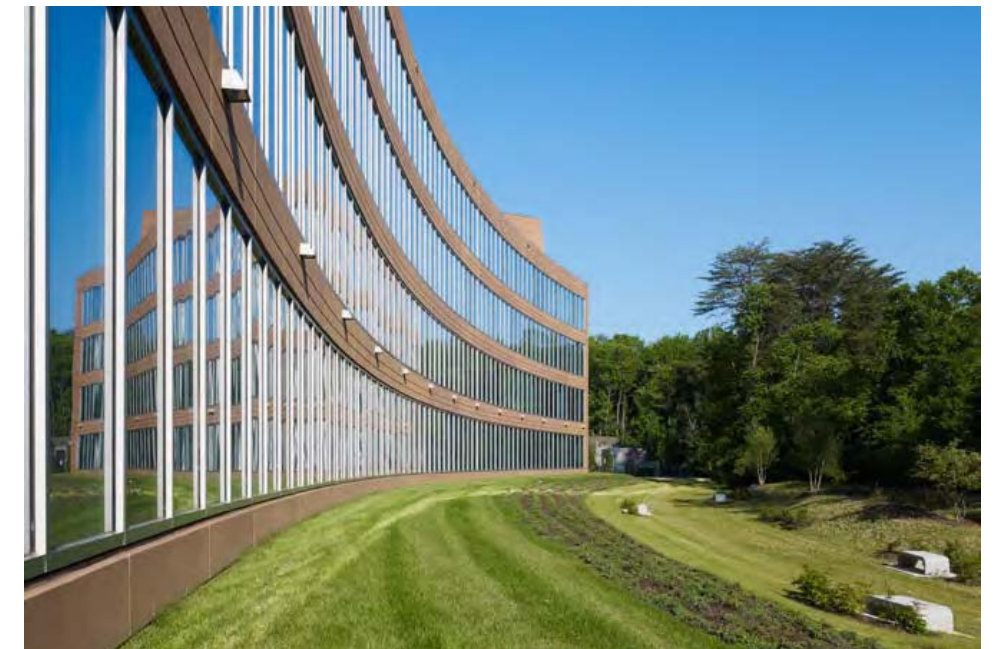
north elevation detail
