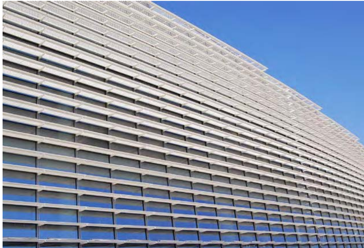
▲ south façade detail
