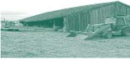
Sod House Ranch Barn Before Restoration USFWS Photo
