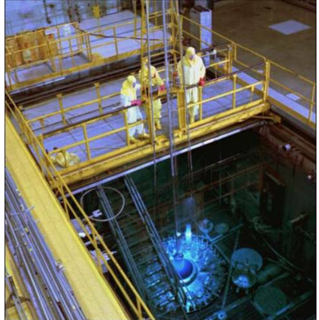
Removal of fuel from the HFIR reactor core.
