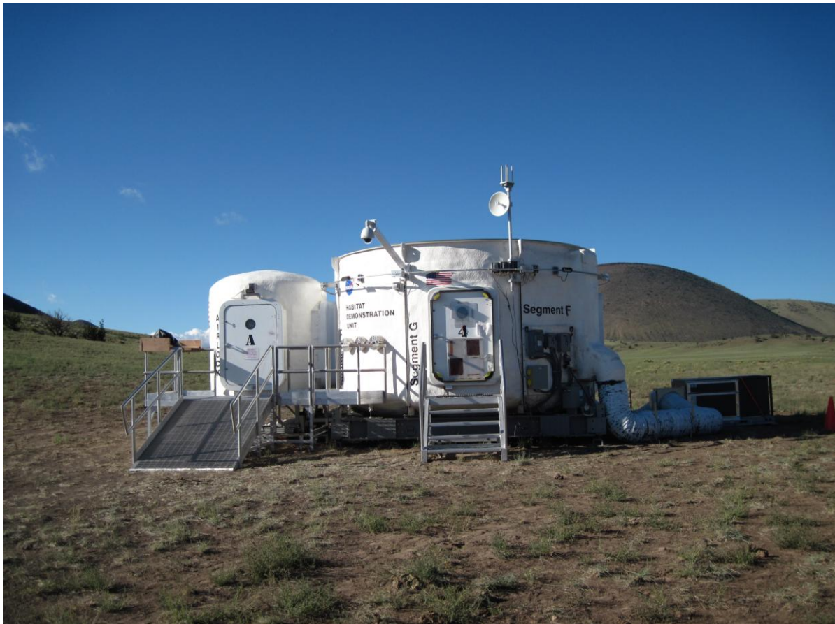
Figure 1.— The HDU in front of the SP Mountain. The large module in the center is the PEM and the smaller structure to the left is the airlock.
