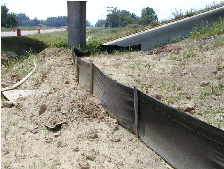
Figure 5-15. Example application of a filter fabric used as a silt fence.
