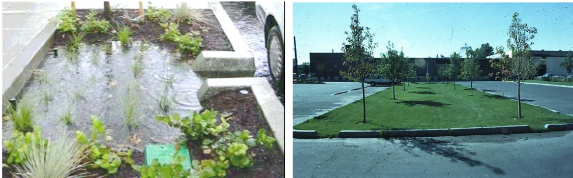
Figure 5-4. Example of Curb Cuts to a Bioretention Cell (left) and Swale (right).
