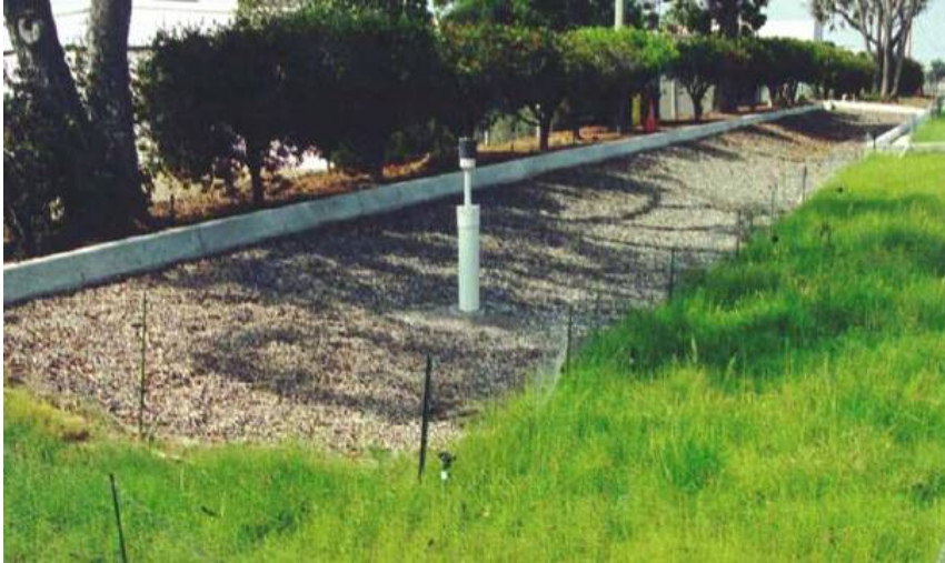
Figure 5-2. Example of an Infiltration Trench Used to Treat Roadway Runoff. Source: California BMP Handbooks ( www.cabmphandbooks.com )
