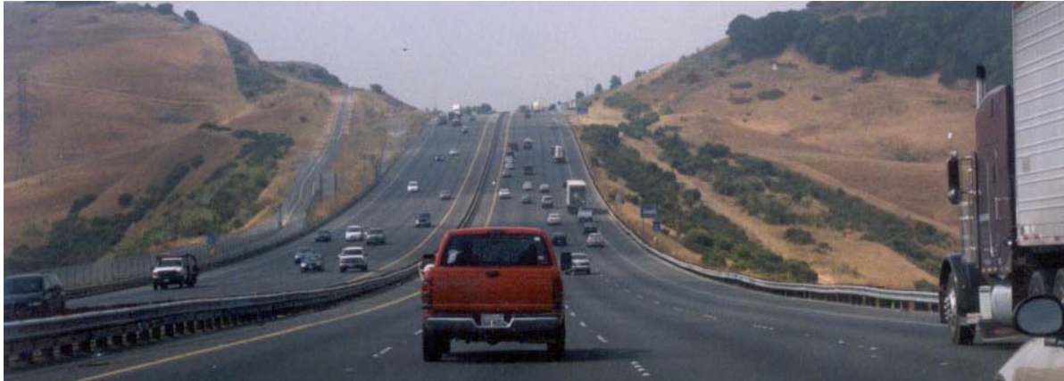
Figure 3-4. Photograph of an Open Drainage System of a Suburban Highway.
