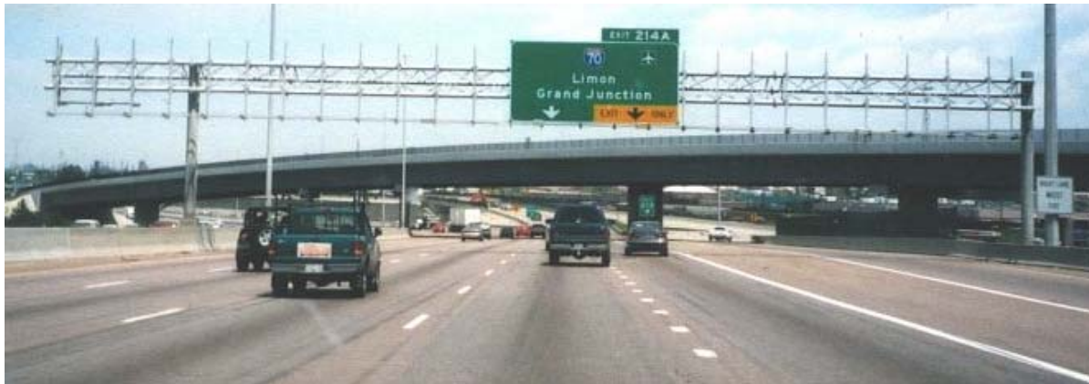
Figure 3-2. Photograph of a Closed Drainage System of an Urban Highway.
