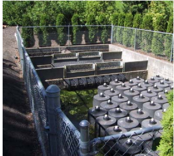
Figure 5-20. Example StormFilter™ Vault
