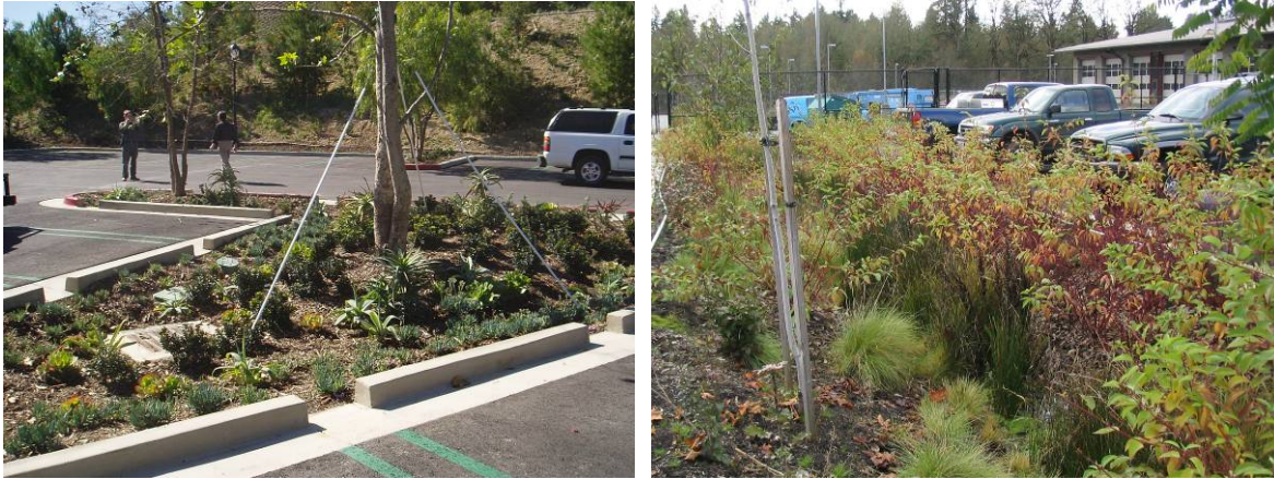
Figure 5-18. Example of parking lot bioretention areas.
