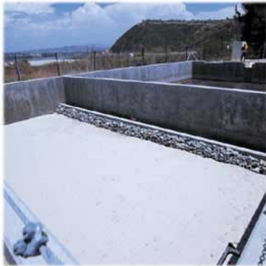
Figure 5-19. Example Austin Sand Filter. http://www.stormh2o.com/images/sw_0103_p67_no.%2012.jpg
