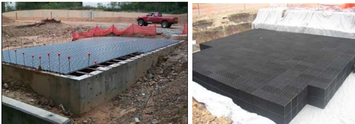
Figure 5-10. Example of Concrete Vault (left) and Modular Storage Tank (right). Source: ARC (2001) and Atlantis (2005).
