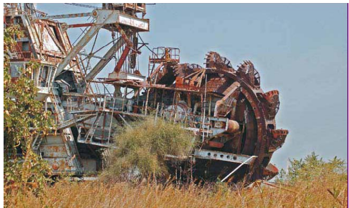
Figure 3-15: Wreckage of the Jonglei Canal Excavator, Testimony to the Risks Associated With Large-Scale Projects in Sensitive Areas
