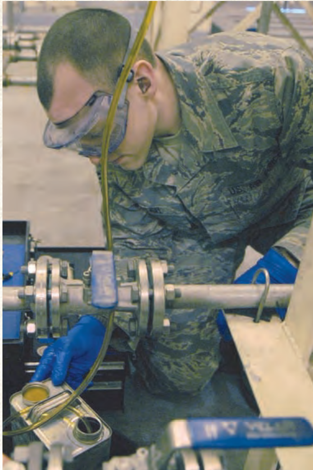
An airman collects a fuel sample at the tanker pump house, Eielson Air Force Base, Alaska. DLA Energy Pacific employees are divided into the Alaska, Guam, Japan and Korea sub-regional offices. Photo by Airman 1st Class Lauren-Taylor Garcia
