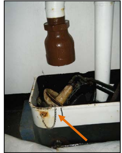
Figure 1: STBD cofferdam (note: plug is not inserted)
