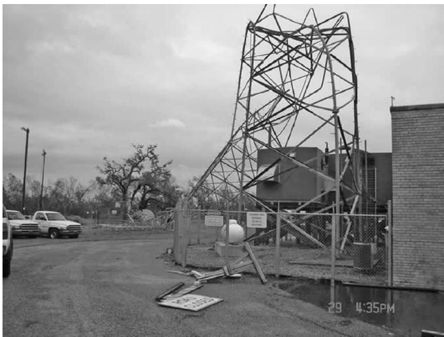
Figure 16-9: Plaquemines Parish (Louisiana) Radio Tower – August 29, 2005
