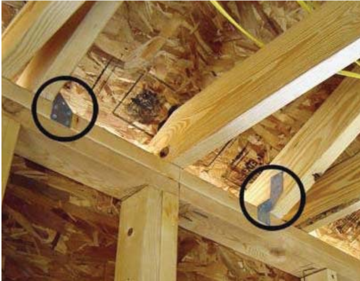
Figure 4. "Hurricane clips" help anchor roofs to prevent detachment due to severe wind.
