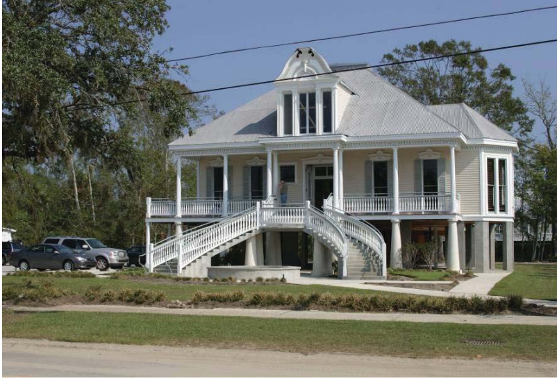
Figure 3. A home in a flood-prone area has been elevated.
