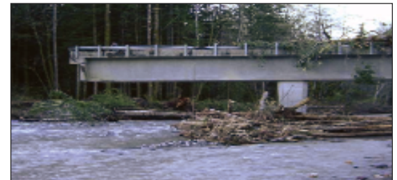
The damage to Boundary Bridge in 2003 will require a new bridge span.
