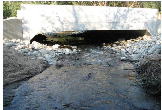
Completed fish passage project
