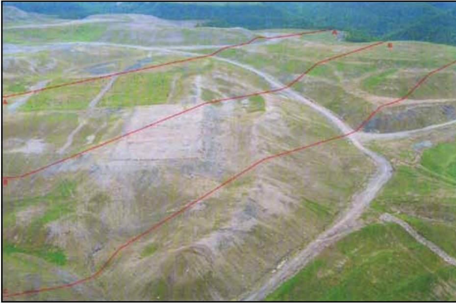
Figure 44: Aerial photograph with GPS generated cross sections.
