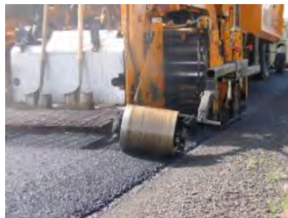
Figure 17. Paver forming and compacting pavement edge treatment.
