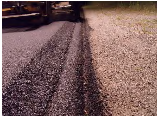
Figure 43. Pavement edge treatment produced by the Advant-Edge™.
