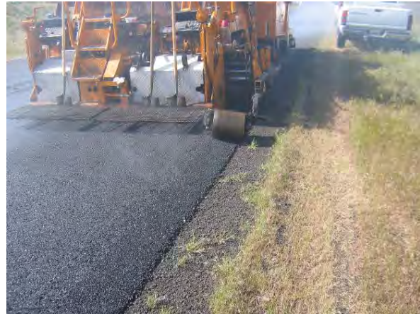
Figure 21. View of rolled pavement edge treatment.
