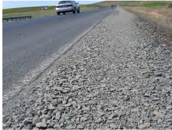
Figure 25. Finished pavement with shoulder material in place.
