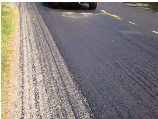
Figure 27. SR 410 prior to construction.
