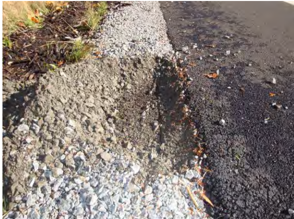
Figure 35. Dig out showing slope of pavement edge.
