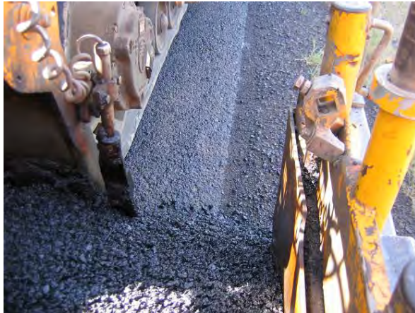
Figure 20. Close-up of sloped pavement edge showing top of slope at existing pavement edge.
