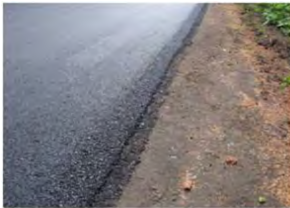
Figure 31. Pavement edge treatment after addition of a roller behind the paver.
