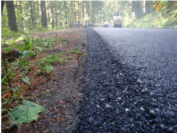
Figure 55. Pavement edge treatment produced by the Carlson end gate.
