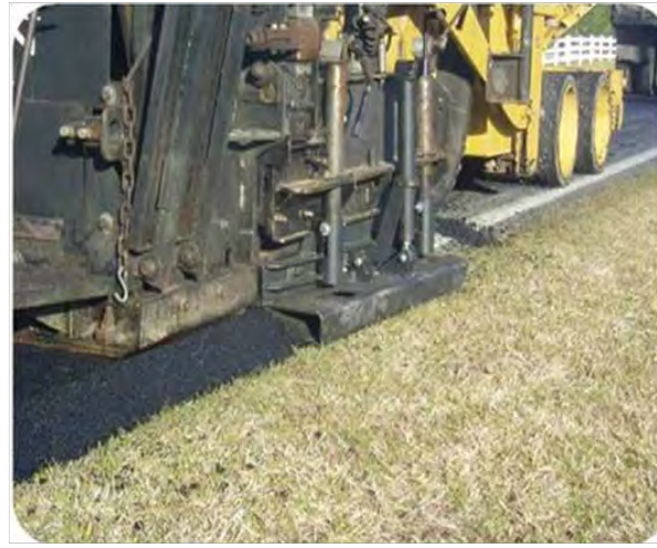
Figure 11. Carlson Safety Edge End Gate in use. (FHWA, Menominee, WI)
