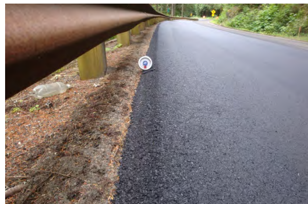
Figure 60. Pavement edge treatment next to guardrail.
