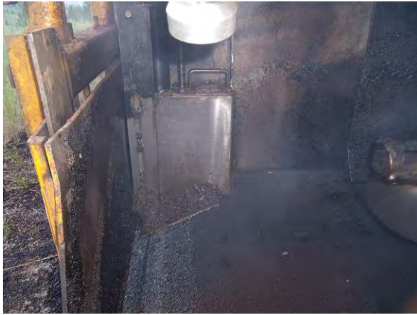
Figure 42. Advant-Edge™ used to produce the pavement edge treatment.
