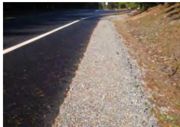
Figure 34. Finished pavement with dressed shoulders.
