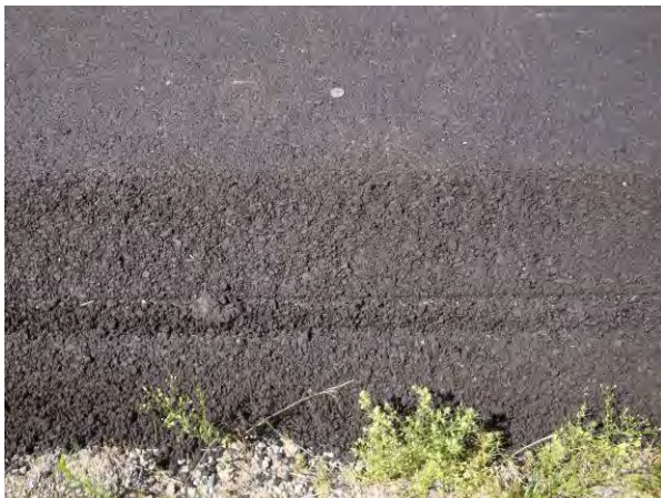
Figure 46. Side view of edge treatment.
