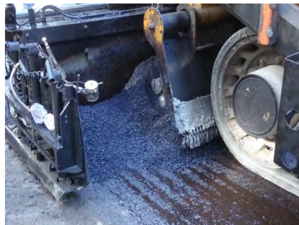
Figure 54. Mix passing through the end gate.
