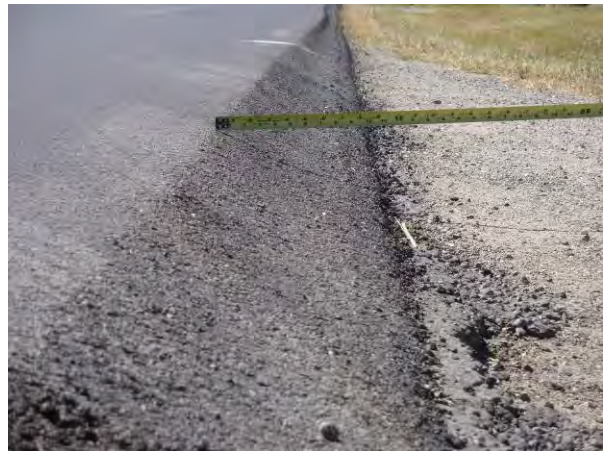
Figure 51. Closer view of slope of edge treatment.
