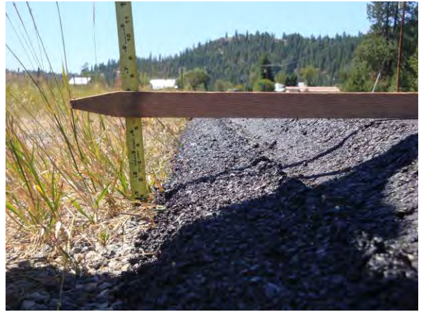
Figure 49. Close-up of edge treatment slope.
