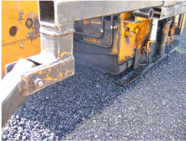
Figure 18. Close-up of paver screed.
