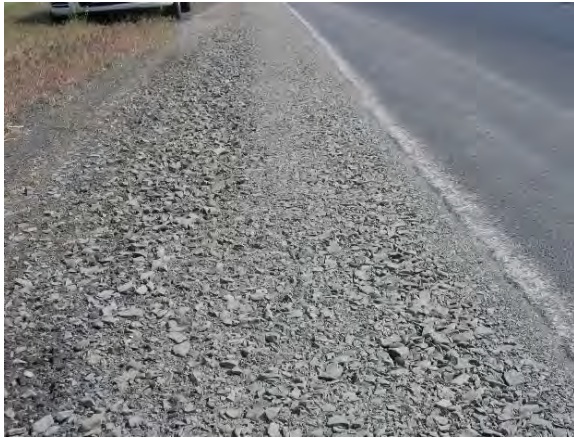
Figure 24. Finished pavement with shoulder material in place.
