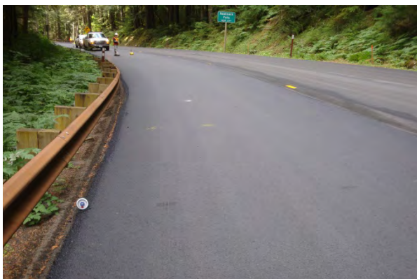
Figure 59. Pavement edge treatment next to guardrail.
