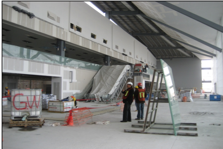
Figure 4.85: General Mariano Escobedo International Airport Terminal B under construction.
