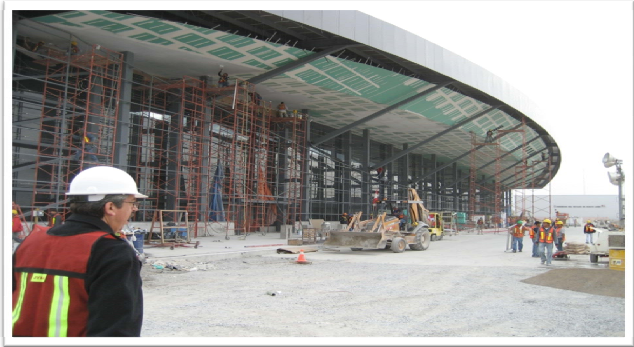
Figure 4.87: Terminal B Construction
