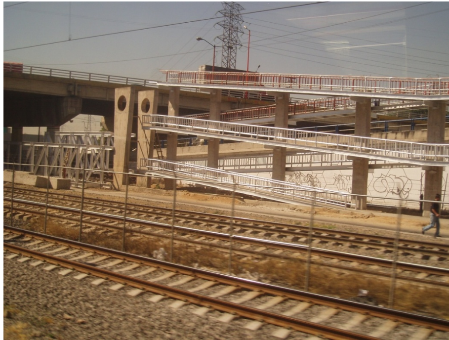
Figure 4.59: Mexico City Commuter Rail Pedestrian Bridges
