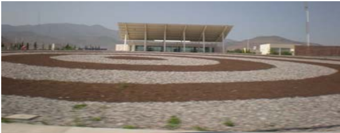
Figure 3.15: San Luis Potosí Industrial Park Customs Zone
