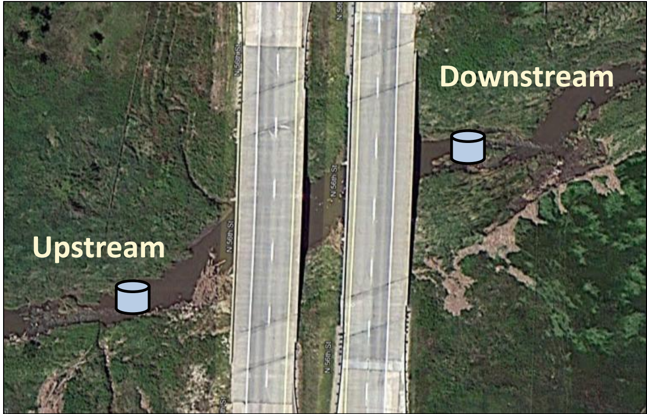
Figure 2.3 Dry weather sampling sites at the Highway 77 over Rock Creek bridge
