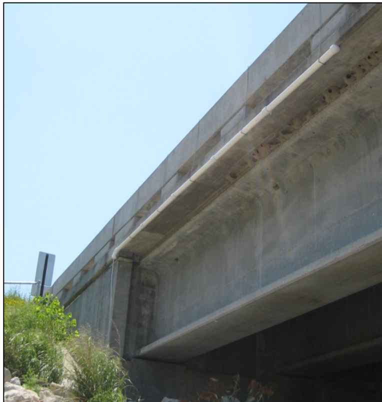
Figure 2.6 Bridge gutter installed at I-80 over Platte River site
