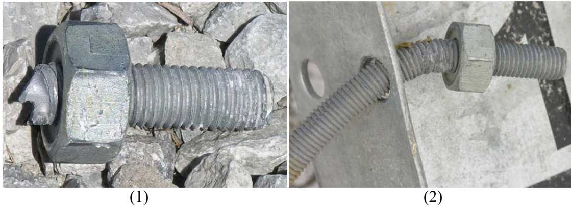
Figure 28. Blockout Bolt Failure Modes
