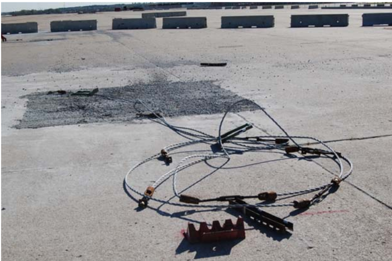
Figure 52. System Damage, Test No. HTCT-1
