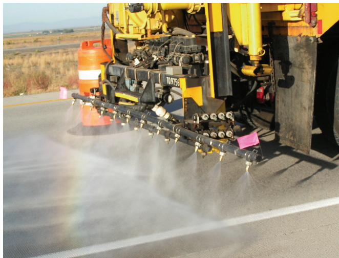
Figure 8.6. Photograph showing topical application of 30%-LiNO 3 solution to concrete pavement in Idaho
