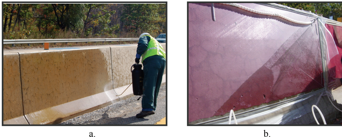
Figure 8.7. Photograph showing topical application (a) and vacuum application (b) of 30%- \text{LiNO}_3 solution to highway barrier in Massachusetts
