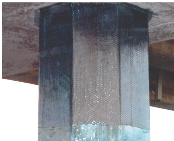
Figure 8.8. Photograph showing typical bridge column wrapped with FRP (Carse 1996)
