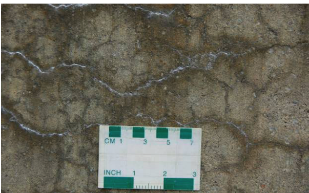
Figure 3.5. (A). Pop-out created by the expansion of a frost-susceptible porous coarse aggregate particle (leached chert). (B). ASR-induced pop-out in a concrete pavement incorporating highly-reactive aggregates; also noted pattern cracking. (C). Efflorescence and exudations of alkali-silica gel at the surface of the concrete foundation of a 25-year-old highway bridge affected by ASR. (D). Efflorescence and exudations of alkali-silica gel at the surface of a small concrete monument affected by ASR. (E). Surface discoloration and exudation associated with cracks.
