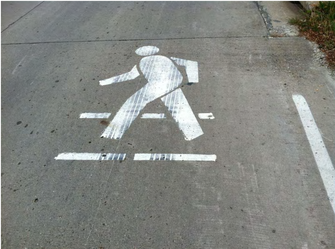
Figure D.16. Pedestrian symbol pavement marking south of North Avenue (County Road G-14) northbound
