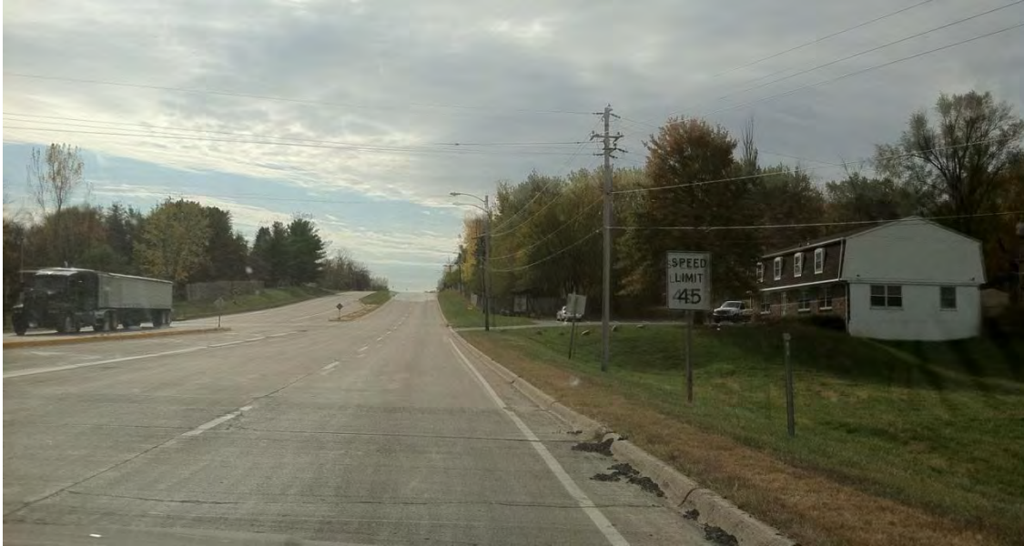
Figure D.15. Approaching Lakewood Drive intersection southbound
