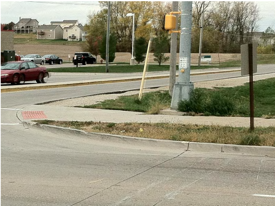
Figure D.18. Northwest radius at the Beardsley Street intersection showing traffic encroachment
