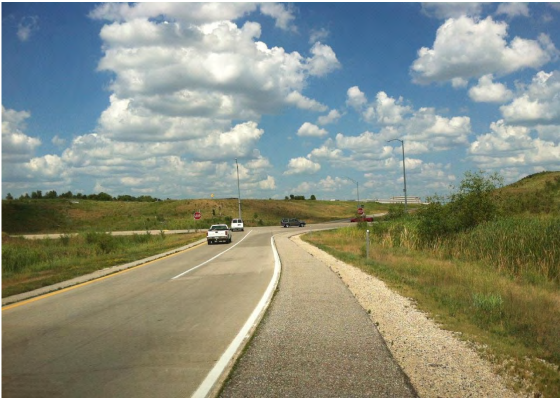
Figure D.22. IA 5 eastbound off ramp approaching IA 28 Stop signs
