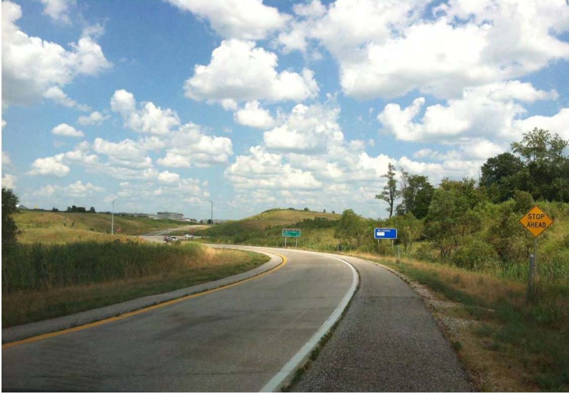
Figure D.21. IA 5 eastbound off ramp approaching IA 28
