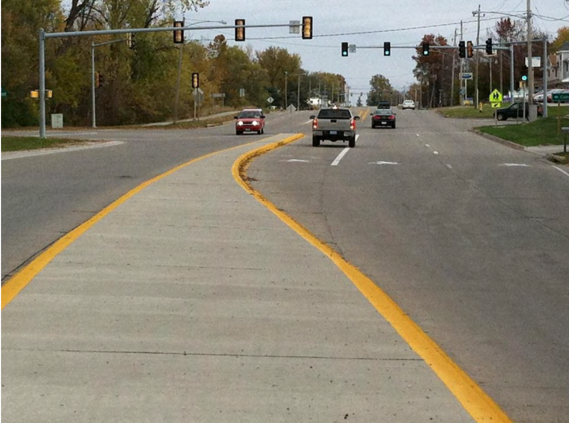
Figure D.1. Approaching North Avenue (County Road G-14) northbound
