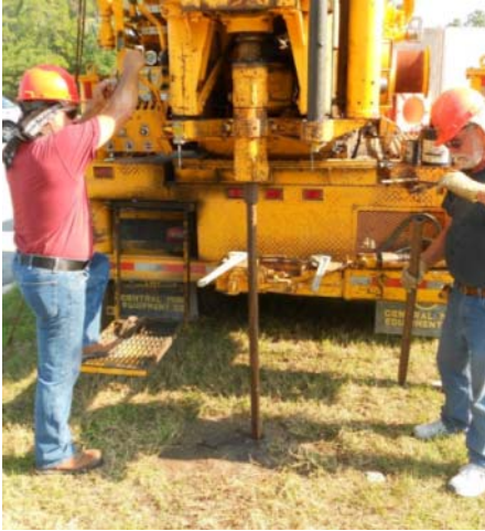
Figure 3-55. Probe being inserted into the ground
