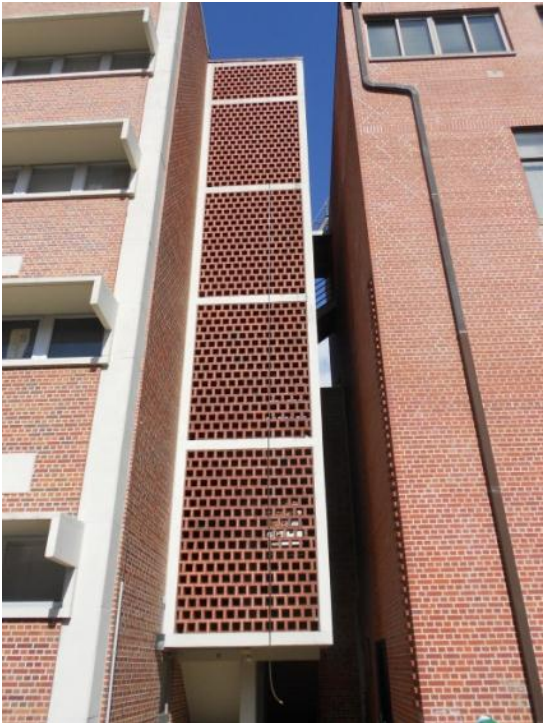
Figure 3-50. Hose attached to falling head vessel hanging from fourth floor of Weil Hall
