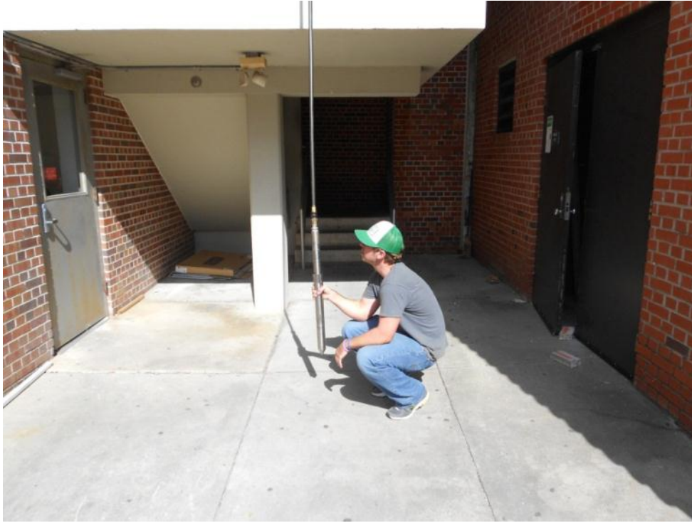
Figure 3-51. Probe attached to hose and monitored for leakage
