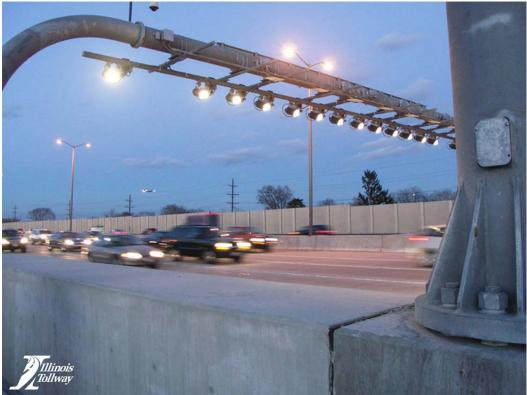
Figure 2-5. A gantry on an open-road tolling system
