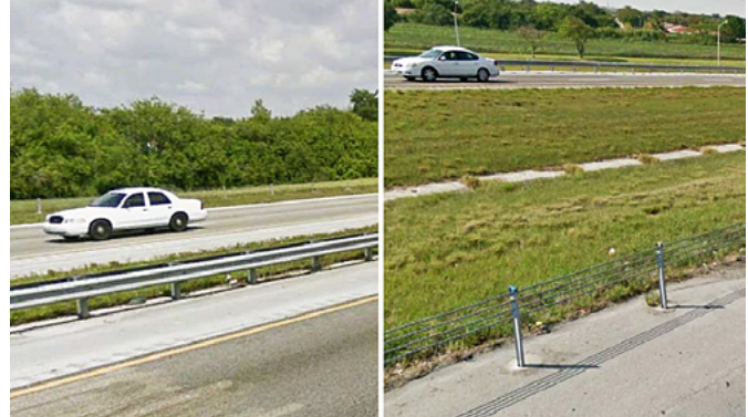
W-beam guardrail (left) and median cable barrier (right) were found to be highly effective in reducing fatal crashes.
