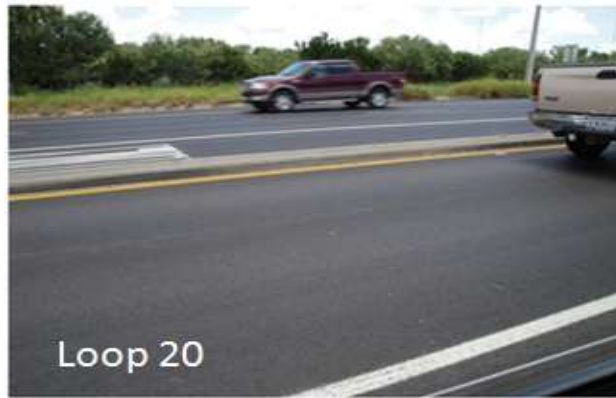
Figure III-3. Example Completed 2" Thick HMA Mats on Loop 20 and US 59. (5.0%PG 64-22 + Crushed Gravel + 20% RAP + 1% Lime)
