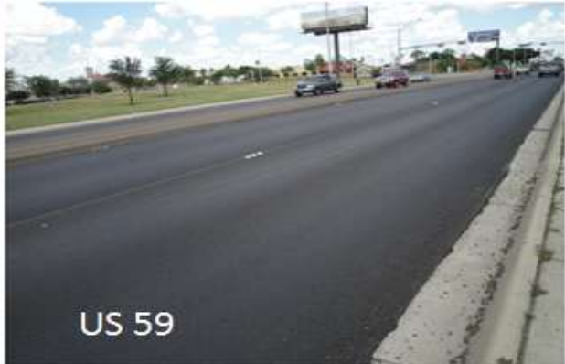
Figure III-3. Example Completed 2" Thick HMA Mats on Loop 20 and US 59. (5.0%PG 64-22 + Crushed Gravel + 20% RAP + 1% Lime)
