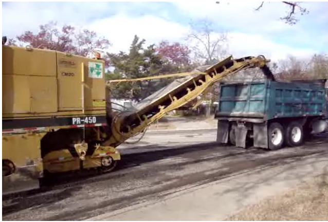
Figure III-1. Example of Milling Operation and Milled-Off section.
