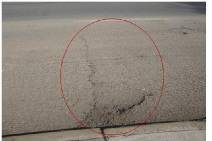
Figure II-3. Example of Cracking on Section 1 - FM 158 EB Intersection of William J. Bryan Pkwy and Pierce St.
