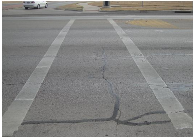
Figure II-1. Example of Cracking on Section 1 - FM 158 WB @ Intersection of Nash Dr. and William J. Bryan Pkwy.
