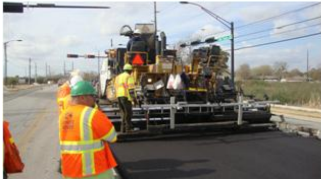
Figure III-3. Paver, IR Bar, and Compactor.
