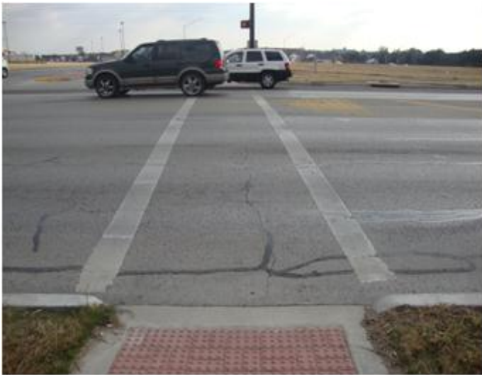
Figure II-1. Example of Cracking on Section 1 - FM 158 WB @ Intersection of Nash Dr. and William J. Bryan Pkwy.
