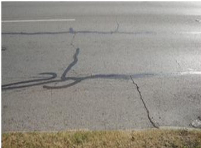
Figure II-2. Example of Cracking on Section 3 - FM 158 WB Adjacent to Brazos County Health Center.
