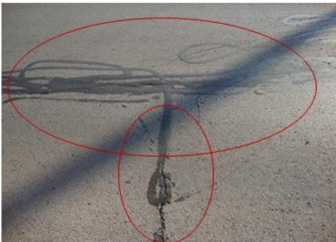
Figure II-3. Example of Cracking on Section 1 - FM 158 EB Intersection of William J. Bryan Pkwy and Pierce St.
