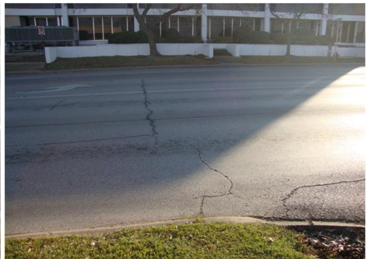
Figure II-2. Example of Cracking on Section 3 - FM 158 WB Adjacent to Brazos County Health Center.
