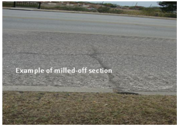
Figure III-1. Example of Milling Operation and Milled-Off section.
