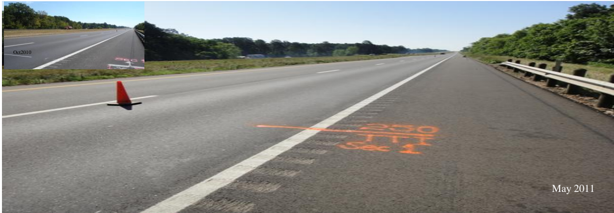
Figure III-1. Test Section 1 (Control: 5.2% Target AC) – No Surface Cracking Observed.
