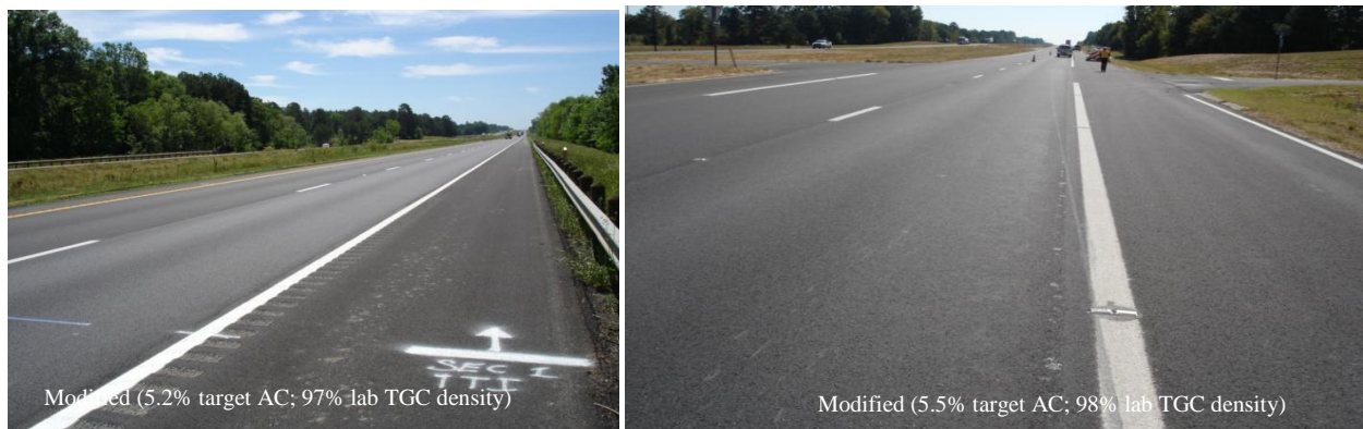
Figure II-2. View of the Test Sections – No Visible Surface Rutting (After 5 Months; Oct 2010).
