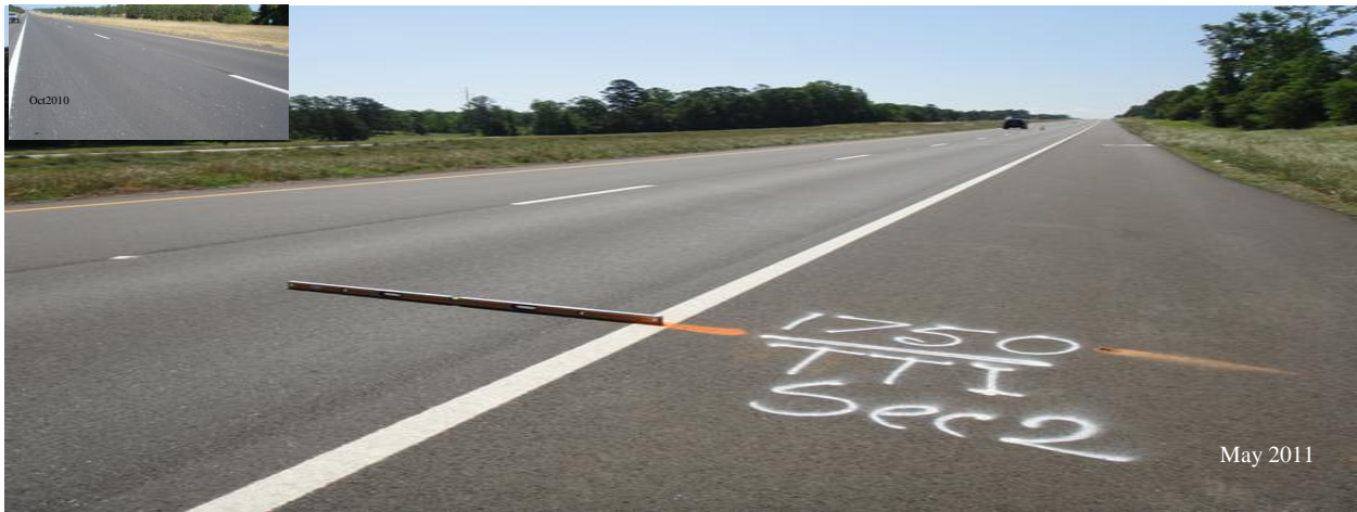
Figure III-2. Test Section 2 (Modified: 5.5% Target AC) – No Surface Cracking Observed.
