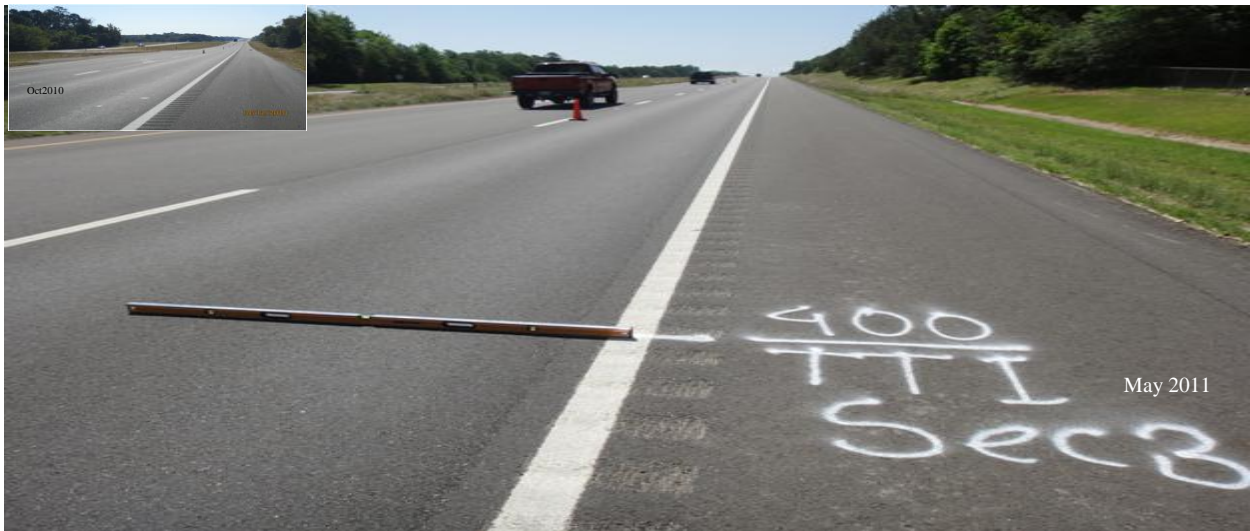
Figure III-3. Test Section 3 (Control: 5.2% Target AC) – No Surface Cracking Observed.
