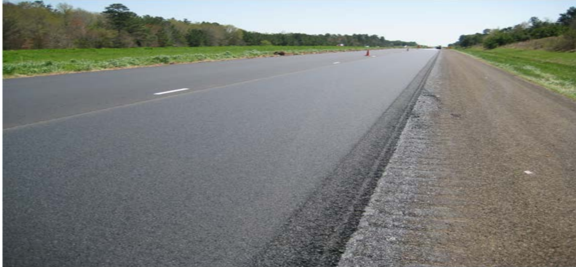
Figure 10. Example of Finished HMA Mat on US 59.
