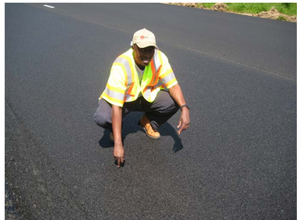
Figure 1f. Example of Finished HMA Mat.
