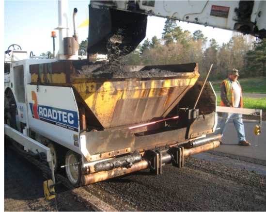
Figure 1b. Roadtec Mixer/Paver.
