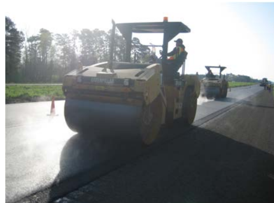
Figure 1d. Caterpillar Vibratory Compactor
