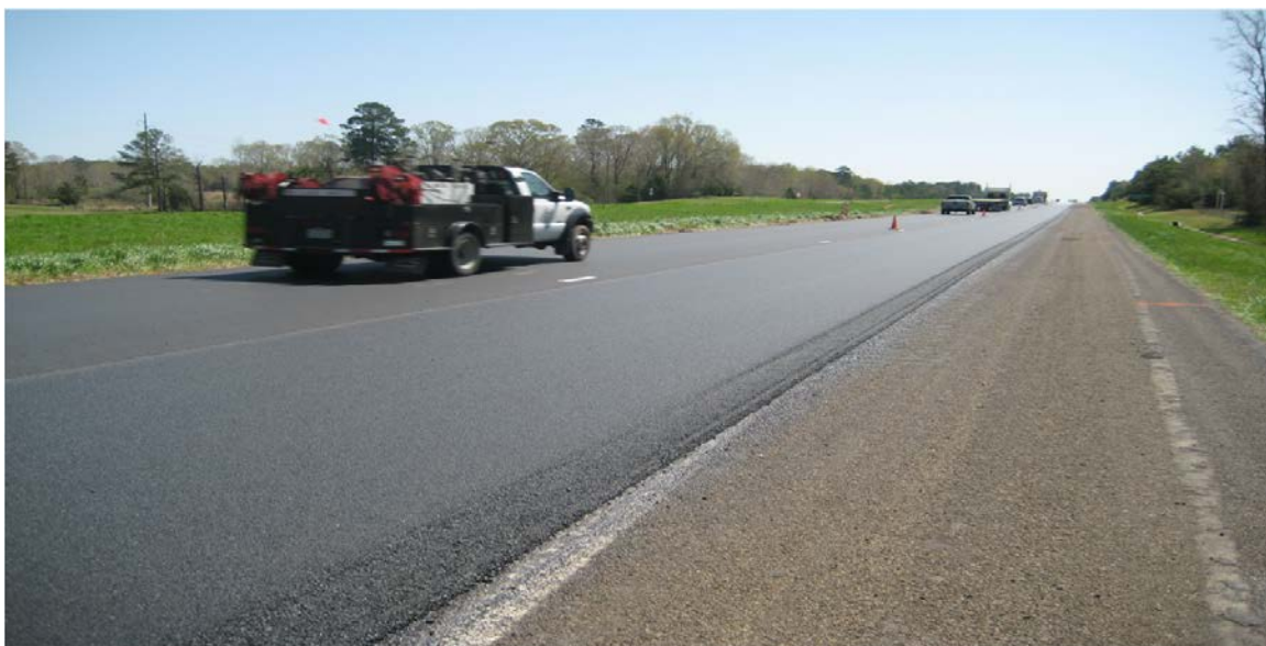
Figure 6. Example of Finished HMA Mat on Modified Section.
