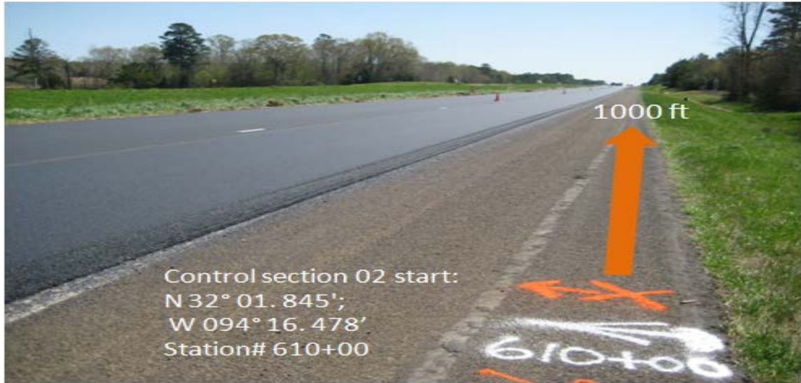
Figure 8. Start Point of TTI Control Section 02.
