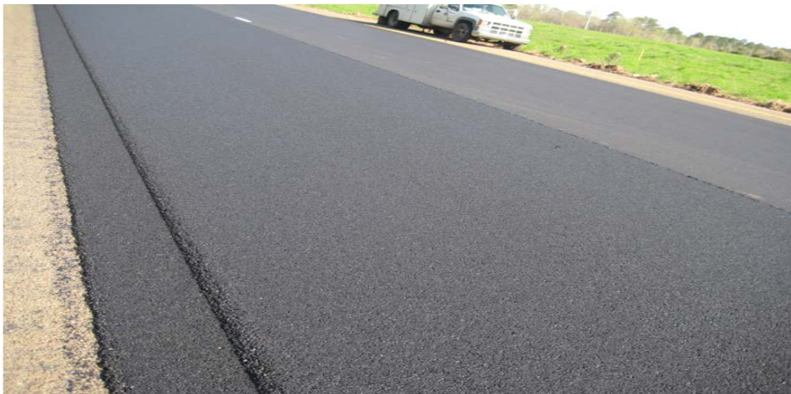
Figure 3. Example of Finished HMA Mat on Control Section 01.
