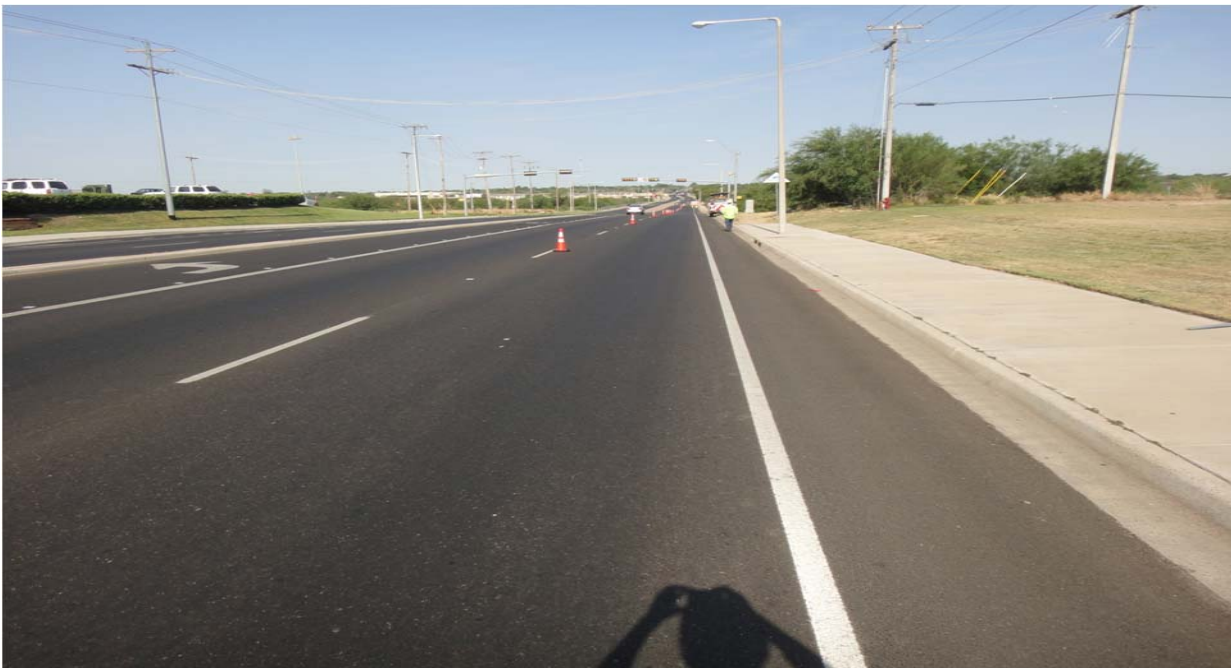
Figure III-2. Spur 400 WB Direction – No Cracking or Rutting Observed.
