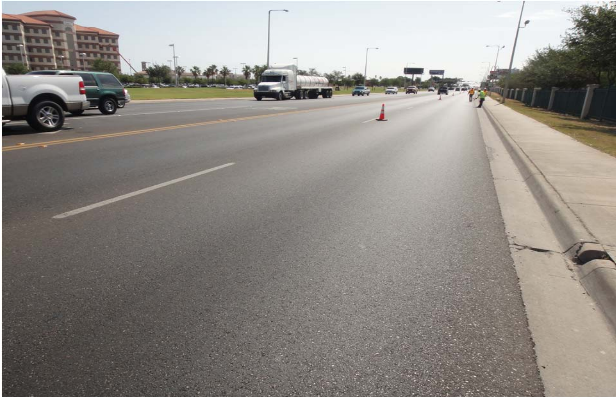
Figure III-3. US 59 EB Direction – No Cracking or Rutting Observed.
