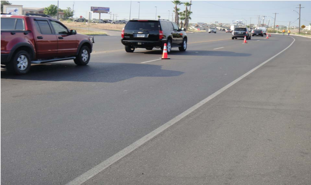
Figure III-1. Loop 20 SB Direction – No Cracking or Rutting Observed.
