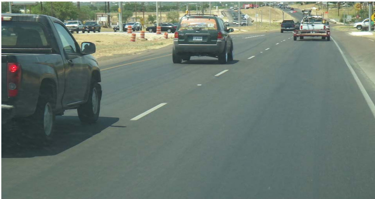
Figure III-4. US 83 SB Direction (Control) – No Cracking or Rutting Observed.
